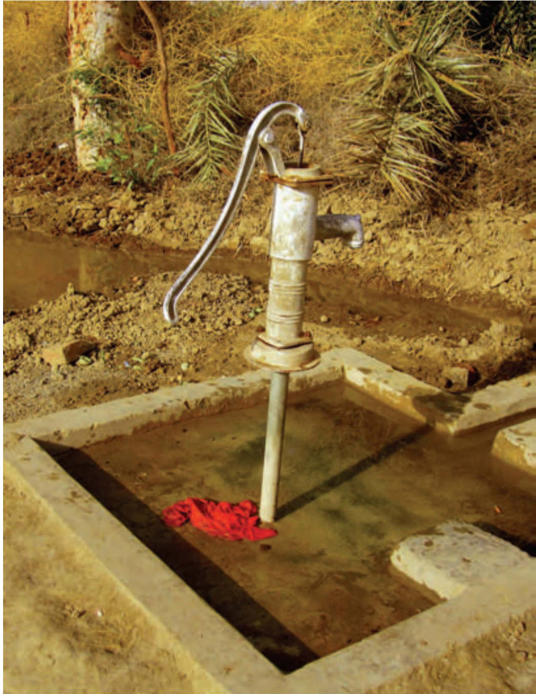
A handpump installed under UCBPRP
